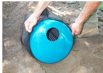
Fig. 62 – Installation of the single offset adapter
