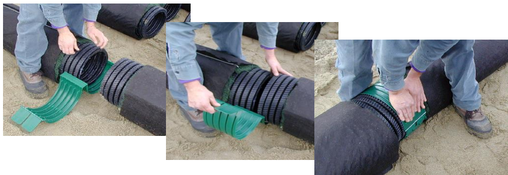
Fig. 60 – Coupling installation
