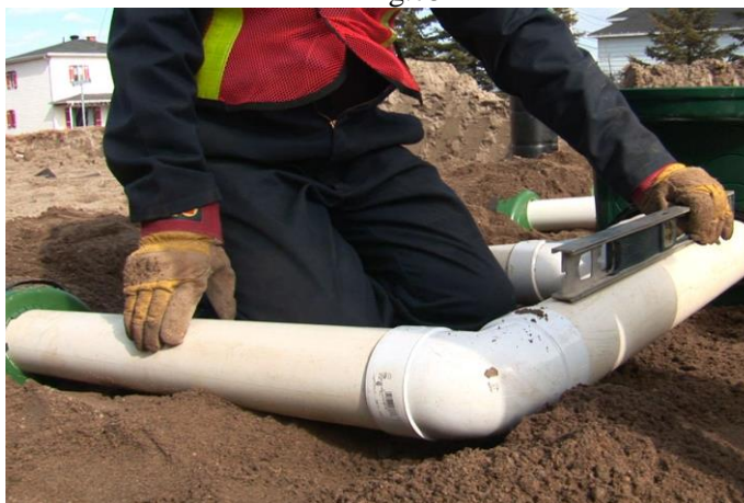
Fig. 76 – Feed Pipe sloped toward Advanced Enviro-Septic ®
