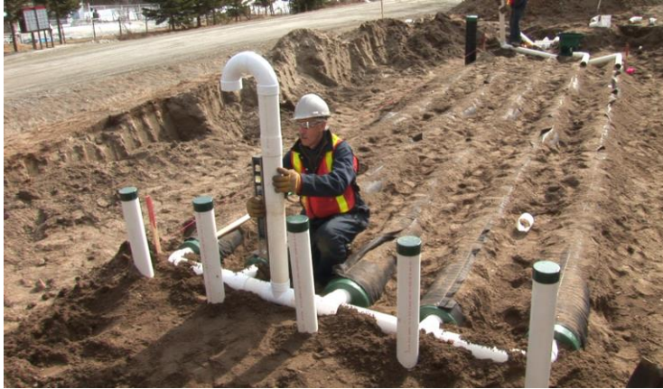
Fig. 69 – Aeration pipe and vent installation
