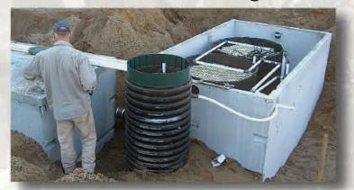
**Basket Biofilter™** systems are completely below ground and can be scaled up for use with any size home. Configured for enhanced Nitrogen removal, Basket systems are ideal for environmentally sensitive areas, high water tables, and clay soils.
