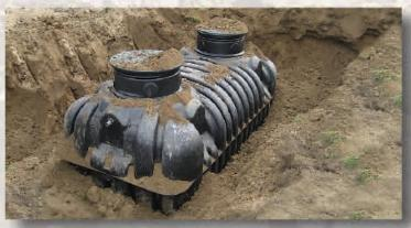
HDPE Tank Biofilters™ are completely below ground, offer enhanced Nitrogen removal, and have a faster and easier installation. These lightweight tanks can be barged to islands, easily maneuvered onto remote sites, and are corrosion resistant in high-sulphur areas.
