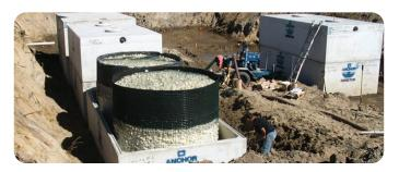
Waterloo Basket Biofilters are constructed of a rigid steel mesh coated for corrosion protection, yet are lightweight and easy to maneuver onsite. Basket Biofilters are placed in locally-available concrete tanks for a completely below ground installation.
