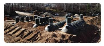
Waterloo Bulk-Filled Tank Biofilters use locally-available concrete or fiberglass tanks that are outfitted as treatment units onsite thereby reducing transportation costs. These completely below-ground installations maximize tankage volume used for treatment reducing the overall footprint.
