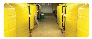
**Waterloo PE-5 Biofilters** are constructed of polyethylene tanks housed in a new or existing maintenance building for year-round use. Highly modular PE-5 Biofilters are ideal for phased-in developments where the wastewater system can expand over time alongside the facility.
