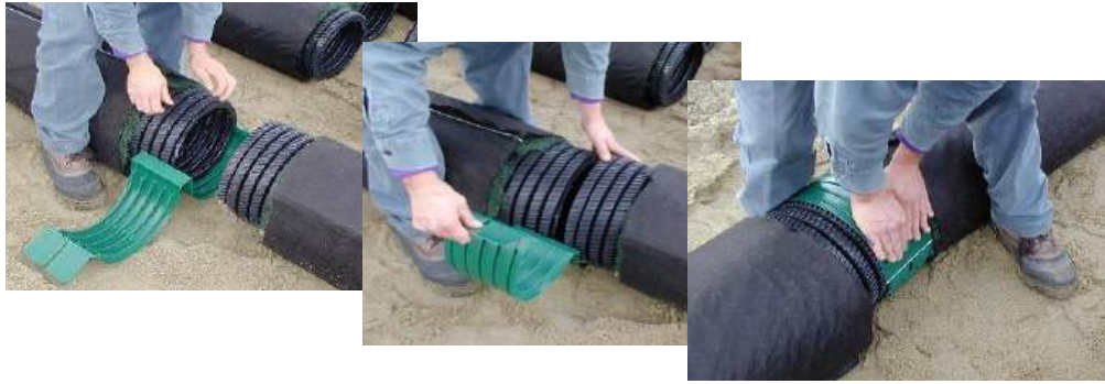
Figure 62. Installation of the couplings
