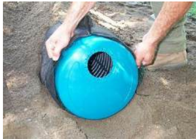
Figure 68. Installation of the Single Offset Adapter
