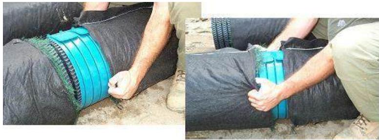
Figure 63. Replacing the geotextile over the couplings
