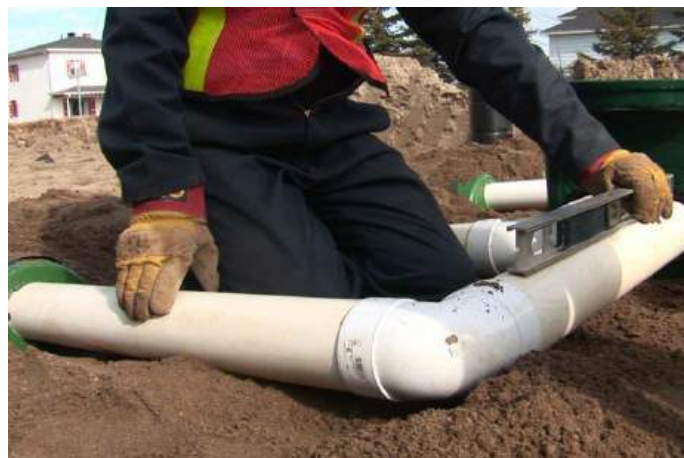
Figure 74. Inlet Pipe sloped toward Advanced Enviro-Septic
