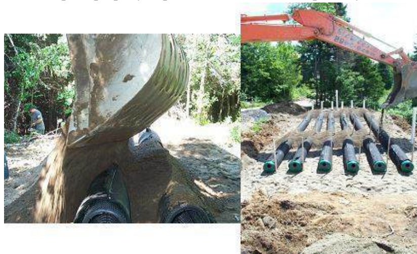
Figure 64. Covering the AES pipes
