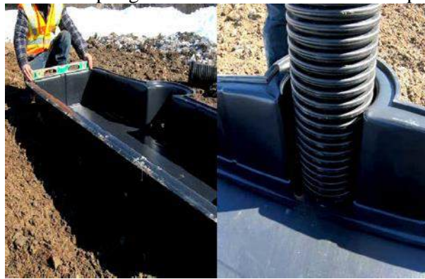
Figure 58. Sampling well installation
